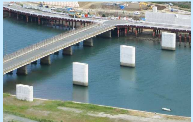
■ Substructure work of Yamato Bridge
